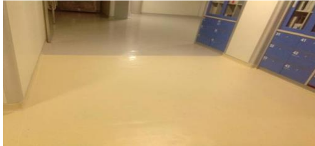
Figure 3. Hospital interior floor walls
