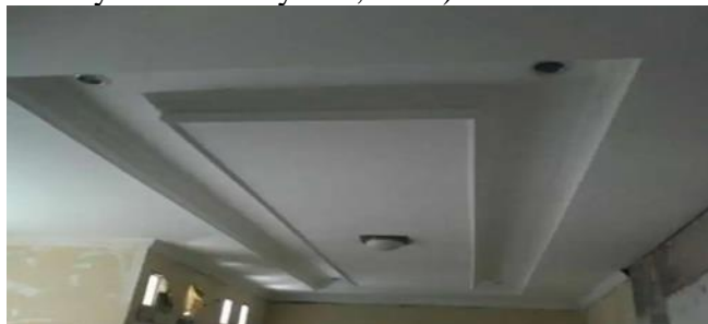
Figure 4. Hospital Interior Ceiling
